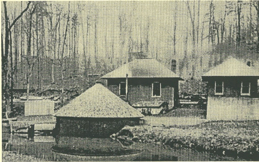
2 The Takoma Park Waterworks on Sligo Creek near Maple Avenue.
