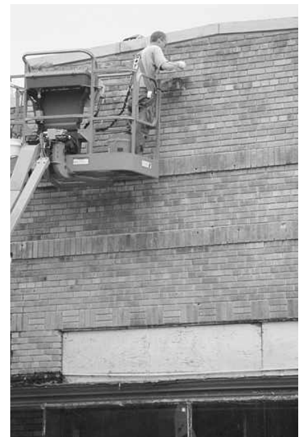
The facade being washed and masonry repointed at 7328 Carroll Avenue by Worcester Eisenbrandt, Inc., a restoration firm based in Baltimore.
