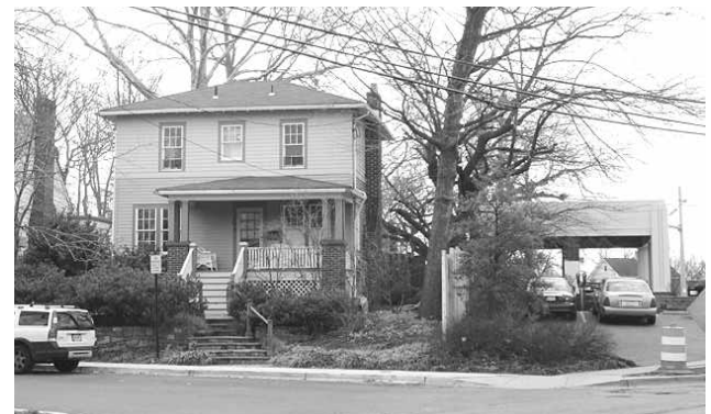
This home will be negatively impacted by the circle.
