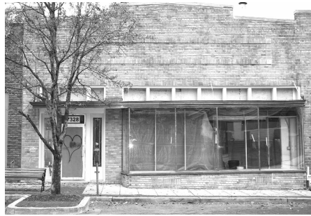
The facade was washed and new glass installed in the bay window of the HTI building.
